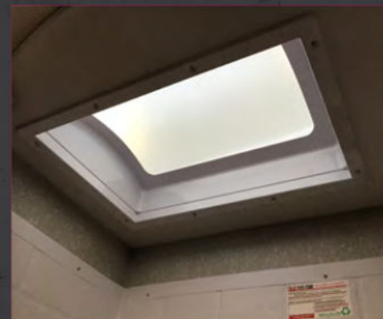
Skylight over Shower
